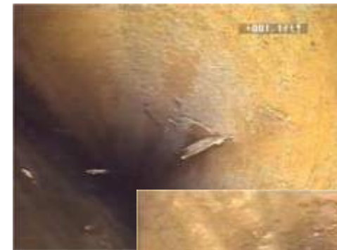
Spalling concrete pipe
