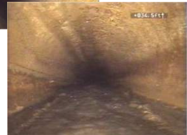
Spalling concrete pipe
