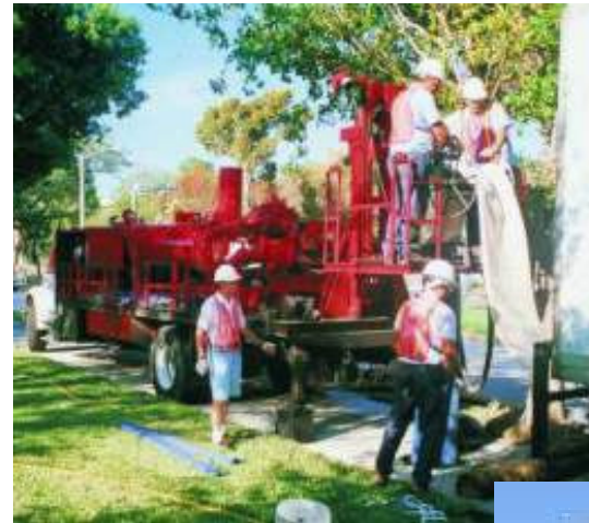
Smaller diameter Installation: Maintaining vehicular and pedestrian traffic
